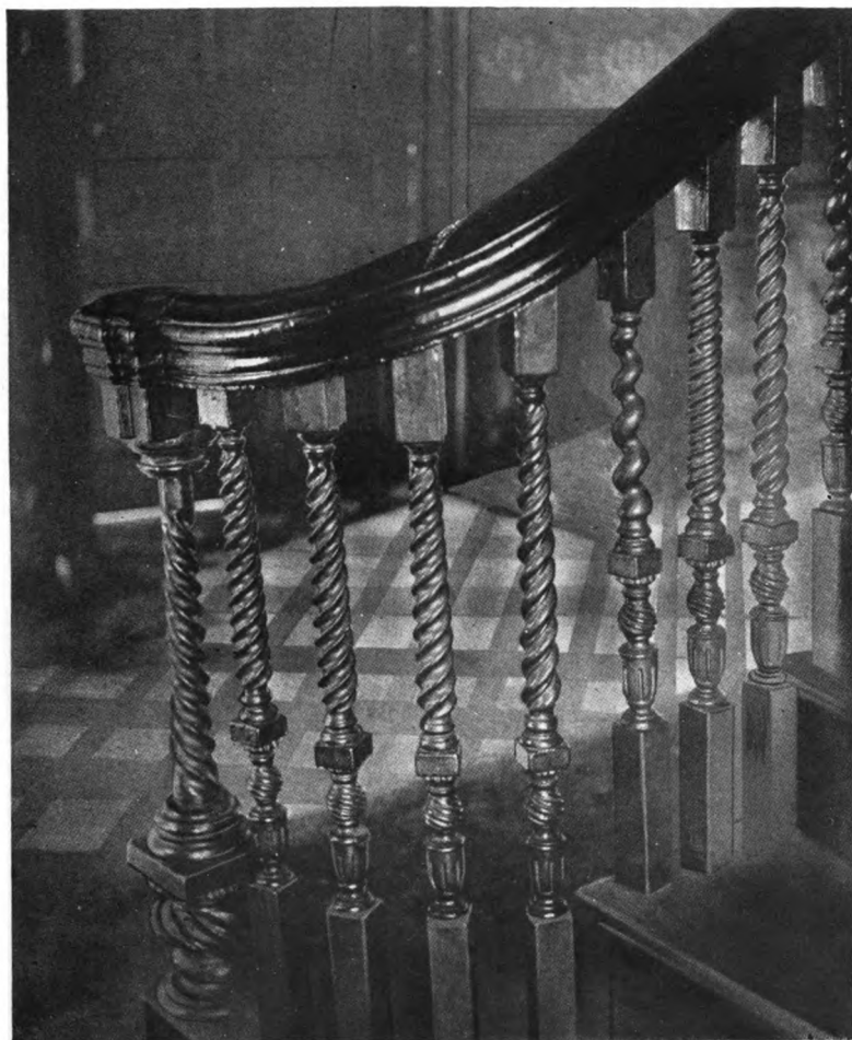
The Historic Staircase, with Mark of Tomahawk on Railing
