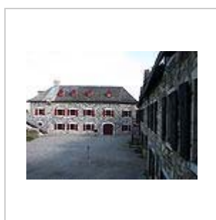
Store room and powder magazine (now Mars Education Center); soldiers' barracks at right
